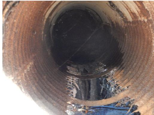
**Photo 10** Near start of Segment B (south end). Existing storm drain outfall proposed for removal and replacement, or daylighting with boardwalk over flow path. 10/26/2015
